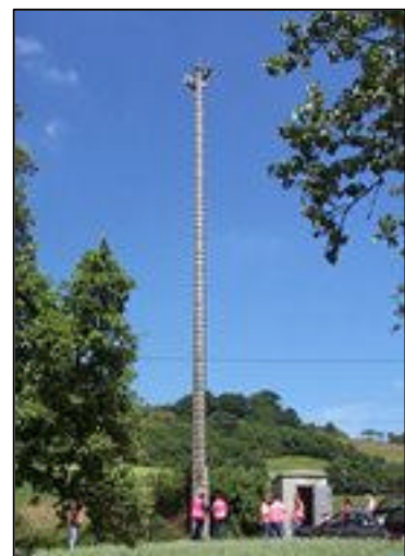
Technical site inspection at an existing mast location
