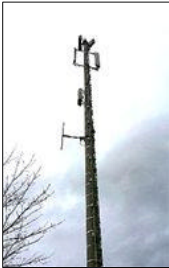
Concrete pole made by centrifugal action
