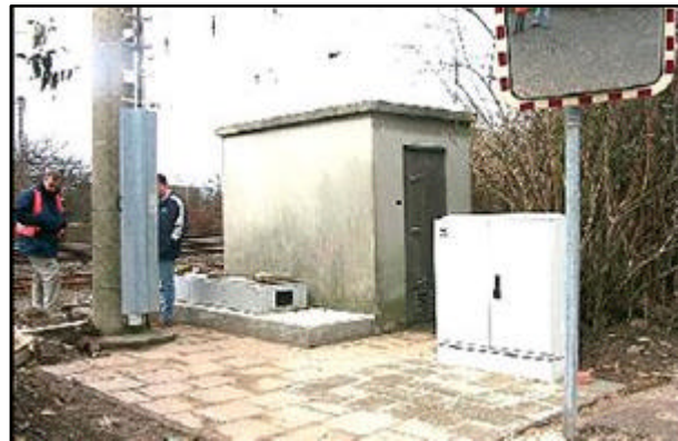
Finished location of a BTS for GSM-R applications
